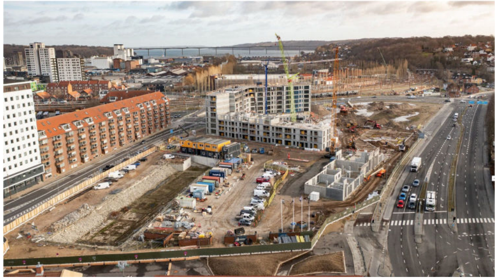
January 2024 – GHV 1+2 and Micro Living under construction
